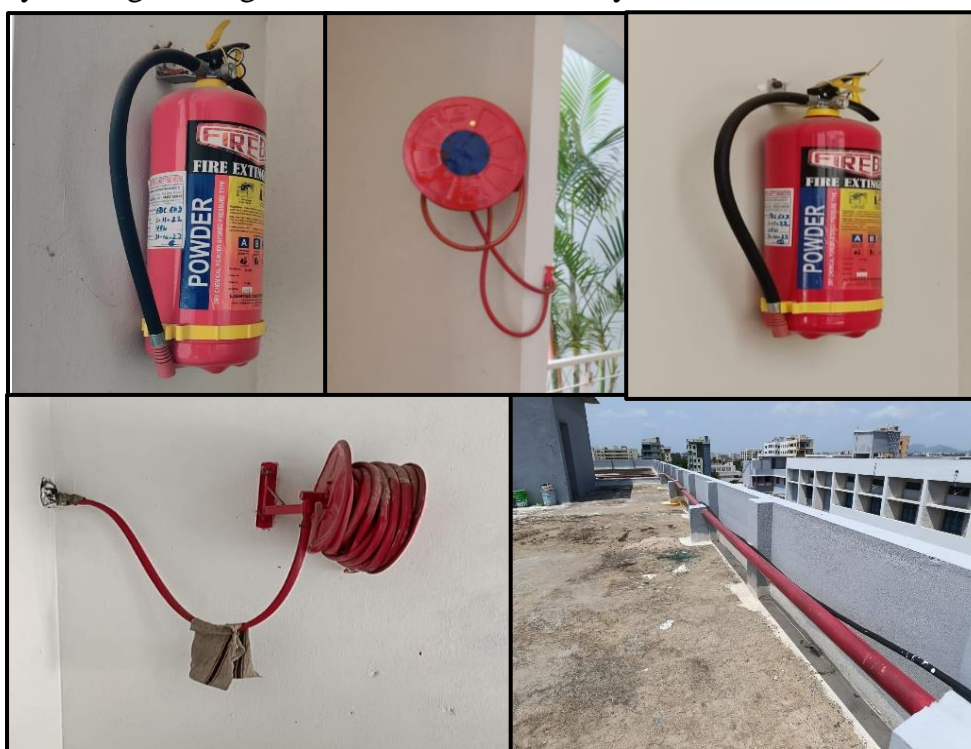
Safety measures in St. Ann's college for women, Guntur, Andhra Pradesh.
